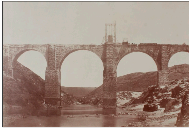
Figure 3. Photograph from downstream during the reconstruction work of the triumphal arch in 1857 after having reconstructed the fifth arch, which had been destroyed [16].
