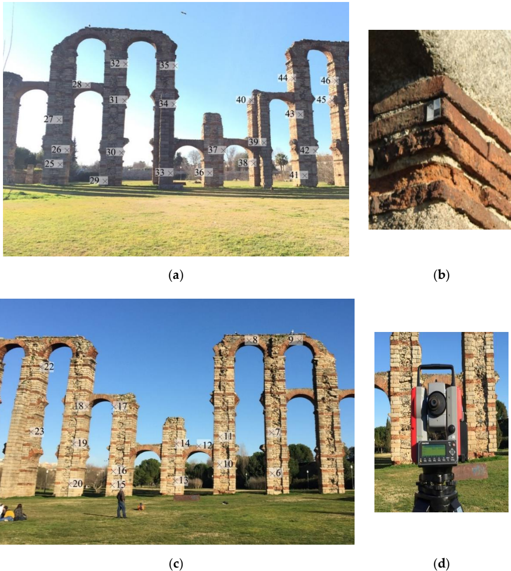
Figure 6. (a,c) Reference points spread on the two fronts of the monument. (b) Target model used in the test and (d) total station Pentax V-227N used to measure the network coordinates.
