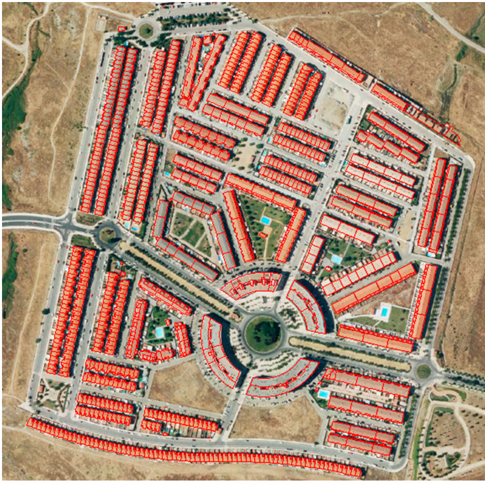
Figure 4. Vector rooftops of a residential part of the city.
