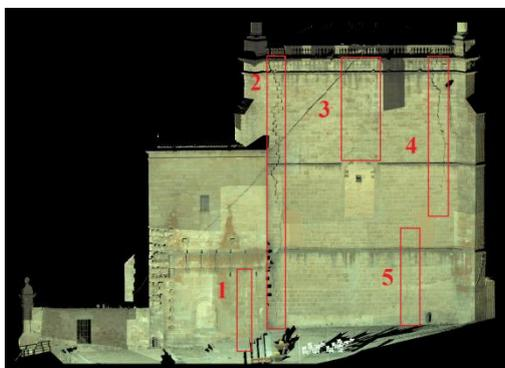
Figure 218.- Cracks in the eastern façade of the cathedral.
