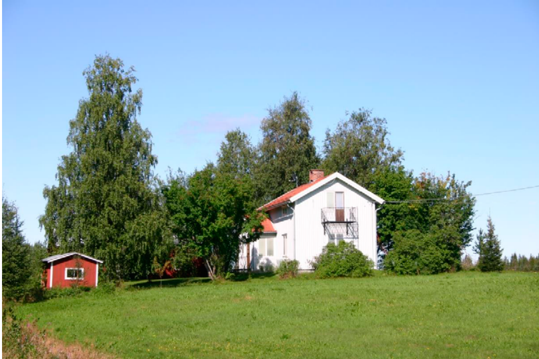
Figure 11. Typical building in the region of Norrland, northern Sweden
