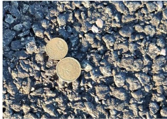
Fig. 2. Details of the road surface.
