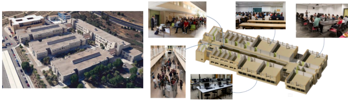
Fig. 2. Exterior and interior views of EPCC: panoramic view, ground floor hall, classroom, meeting room, first floor hall and laboratory (from left to right and from top to bottom).
