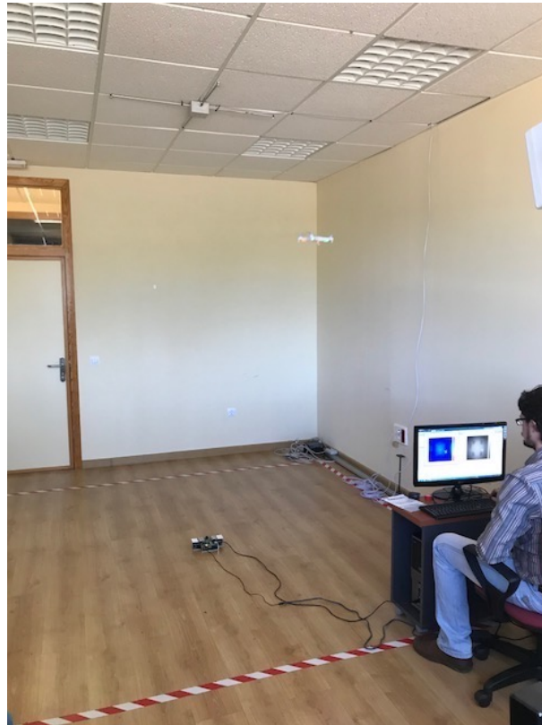
Figure 9. Snapshot of the experimental site, with the ULPS installed in the ceiling of an office room and the TOF-camera placed at the origin of coordinates.
