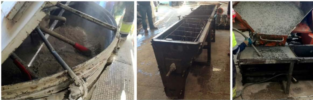
Figure 2. Precast element manufacturing sequence.
