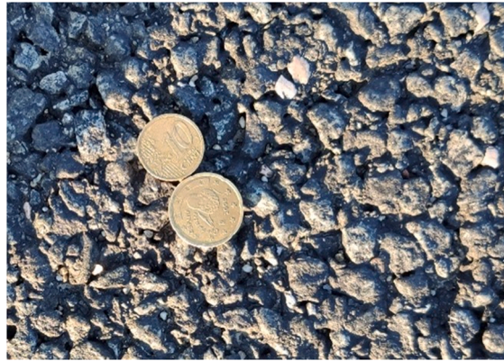
Fig. 2. Details of the road surface.
