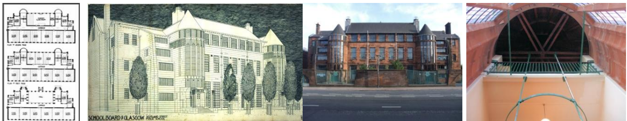
34-37. Scotland Street School. 1905. Glasgow.
